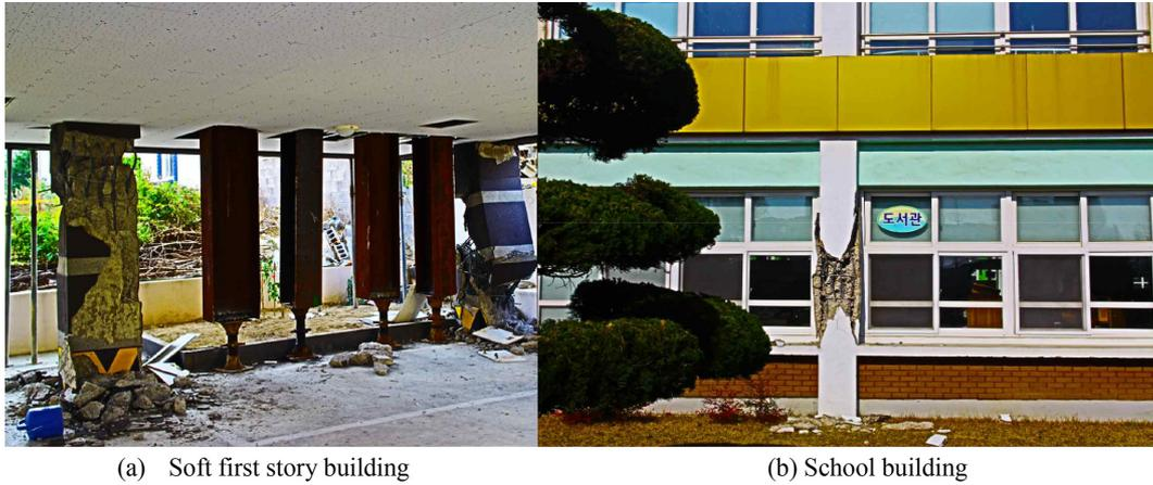
**Figure 1.** Building damage during 2017 Pohang earthquake.
