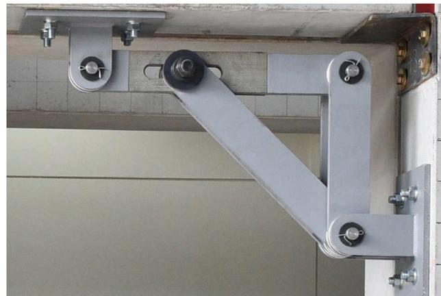
(a) Friction damper (FD) installed at the corner of the PC frame.
