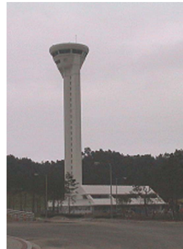
Fig. 4. Control tower of the Yang-Yang International Airport, Korea.
